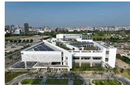
The new E&M and HVAC of China Medical University Hospital
