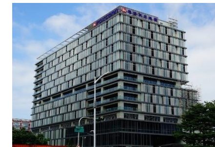
E&M and HVAC of in Kaohsiung Software Park Incubator of Foxconn
