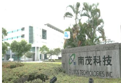
ChipMOS Cleanroom ISO Class 6 construction project 43,110 ft 2
