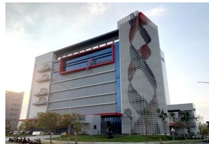
New plant air conditioning of EirGenix
