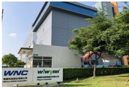
Wiwynn Nanke Factory 1F2F expansion project
