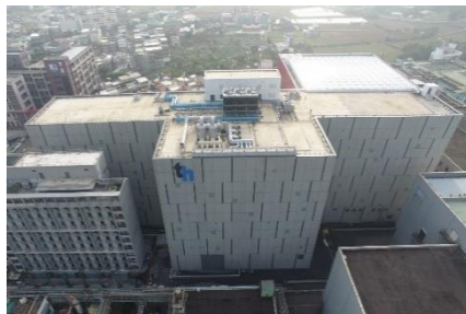
Clean room construction project of TONG HSING
