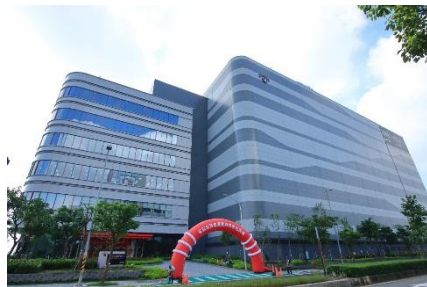
MEP new project in Zhuke Longtan Park of VisEra
